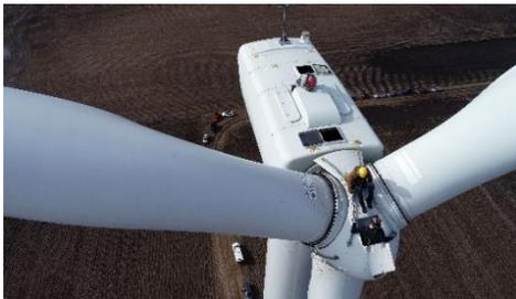
*Wind energy technicians* who inspect and repair wind turbines, another form of renewable energy on the rise. Technicians climb the wind turbine towers to perform maintenance, as well as test electrical, mechanical, and hydraulic components. [Photo source](#).
