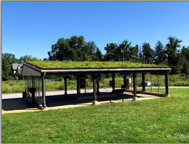
The Green Roof at Duke also has two demonstration rain barrels, which help collect rainwater that can be utilized in gardening and many other outdoor activities.
