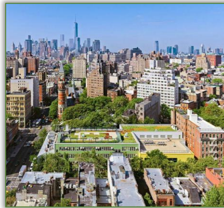
Public School 41 in Greenwich Village, NYC boasts an expansive green roof!
