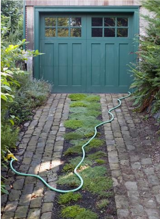
Eco-friendly green driveways – A living permeable driveway, porous and alive – reduce storm drain run off with a rustic look. Photo source: Chic Ecologist
