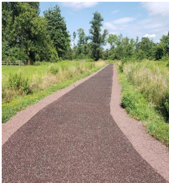
Permeable pedestrian path at Duke Farms.
